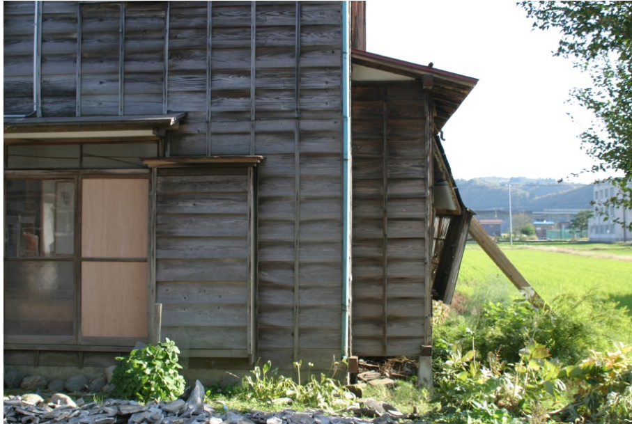
Photo 1: Damaged house in Kawaguchi town
