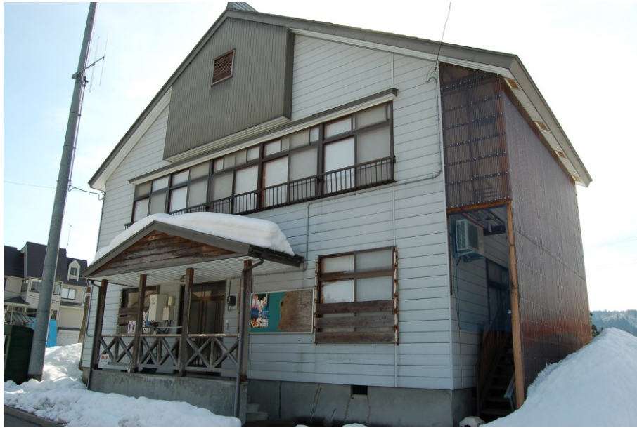
Photo 3: Typical community driven emergency sheltering house in Kawaguchi town
