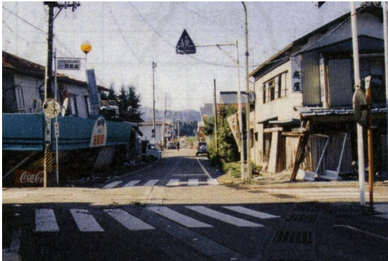
After the earthquake
