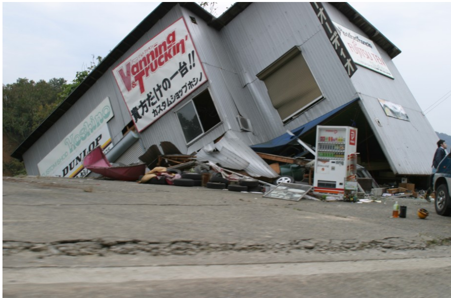
Photo 2: Heavily damaged shop and roads in Kawaguchi town
