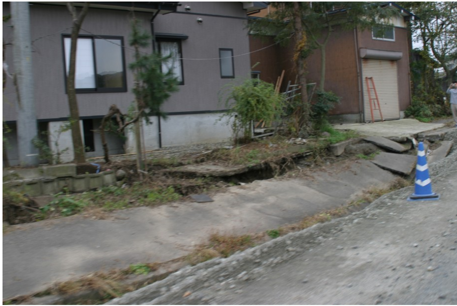
Photo 3: Road damages in Kawaguchi town
