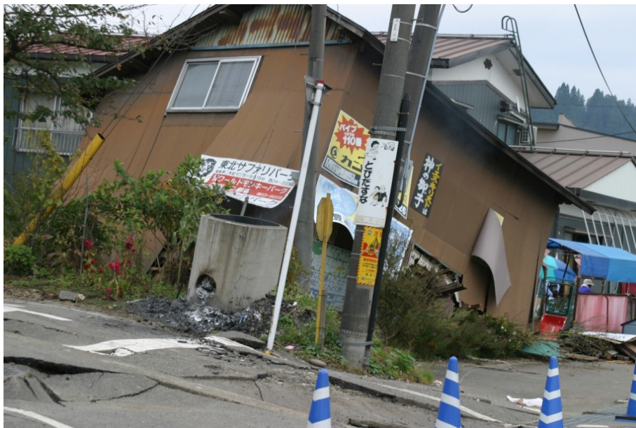
Photo 4: Heavily damaged houses in Kawaguchi town
